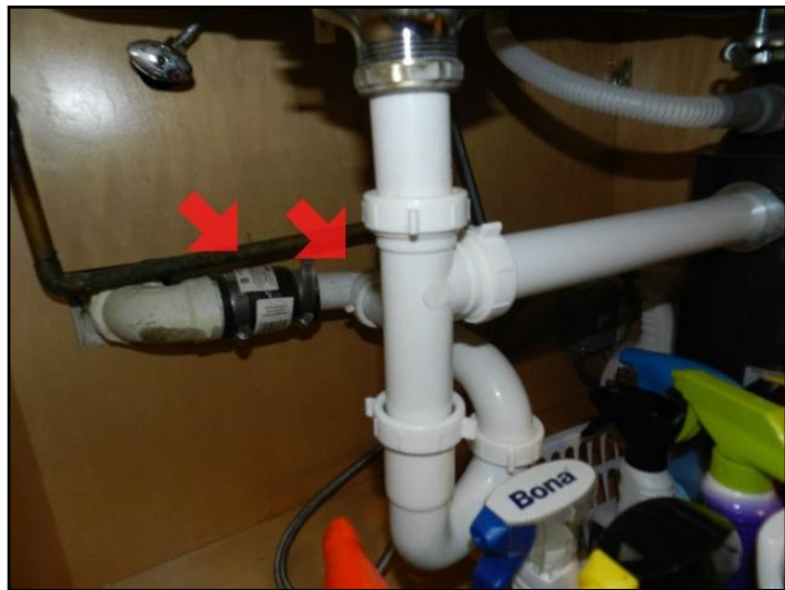
78. Negative slope to drain, PVC piping
