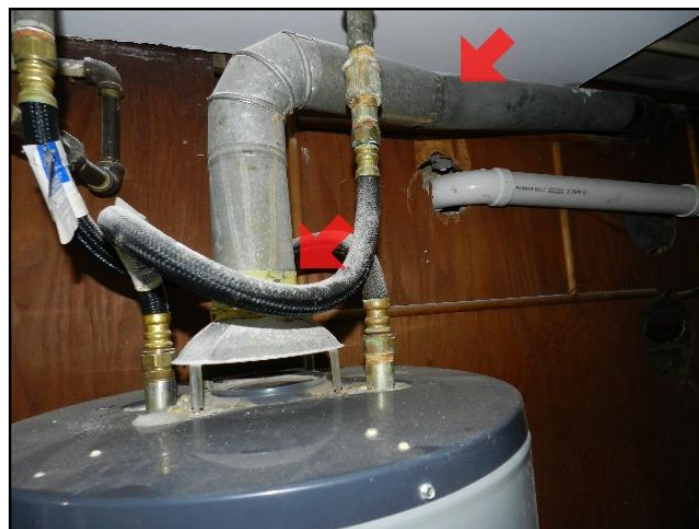
77. Poor connections
