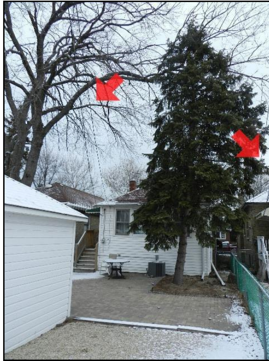
39. Branches / vines interfering with wires
