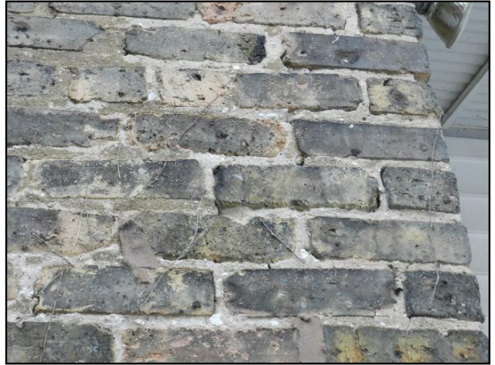
10. Masonry deterioration
