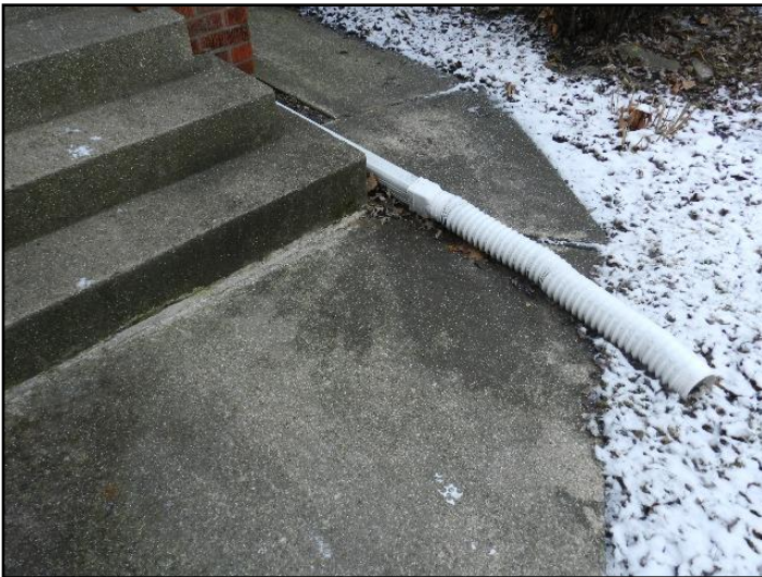
6. Tripping hazard, loose or damaged
