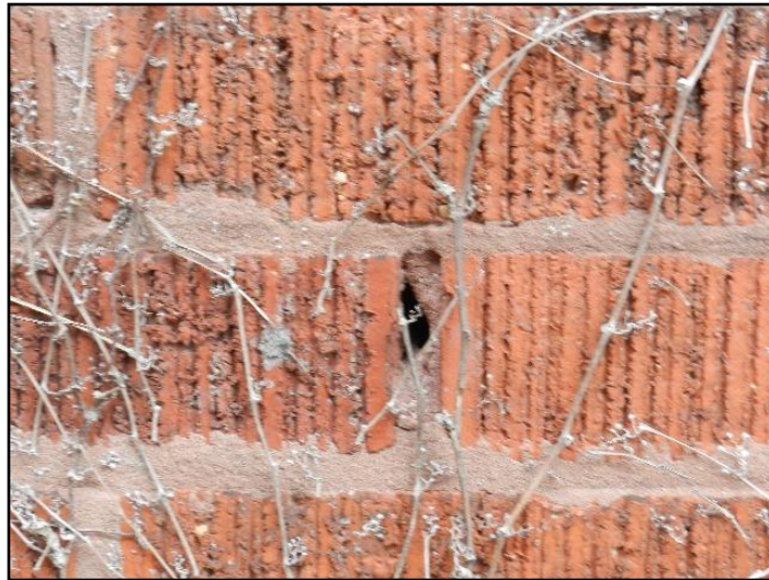
13. Mortar deterioration
