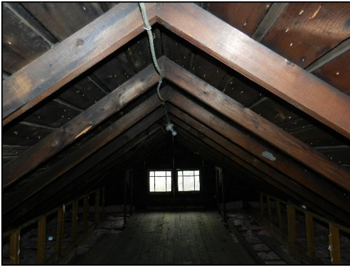
36. No ridge beam, no collar ties
