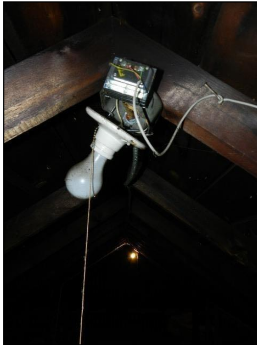
48. For junction box is loose
