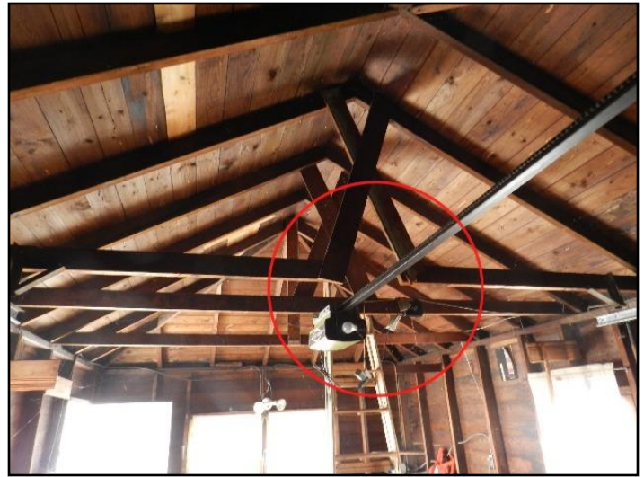
37. Cut roof framing joists
