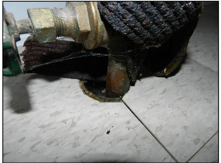
117. Loose floor tiles
