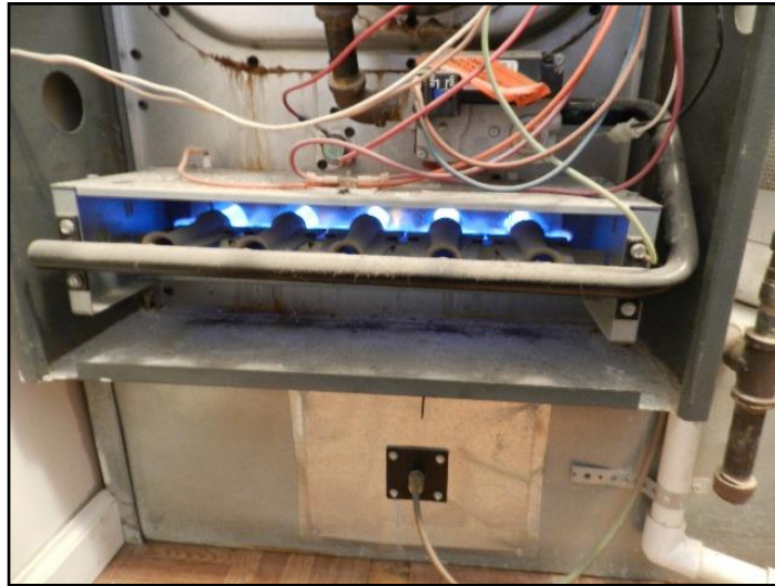
71. Poor flame color or pattern
