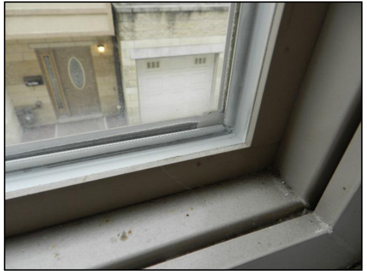
25. Lost seal on double or triple glazing
