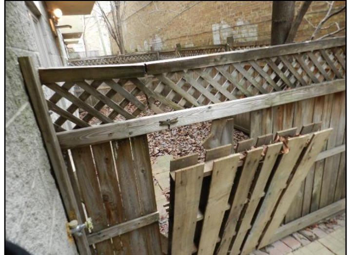
38. Boards damaged
