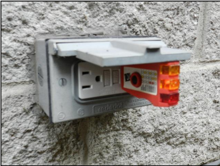
66. Reversed polarity
