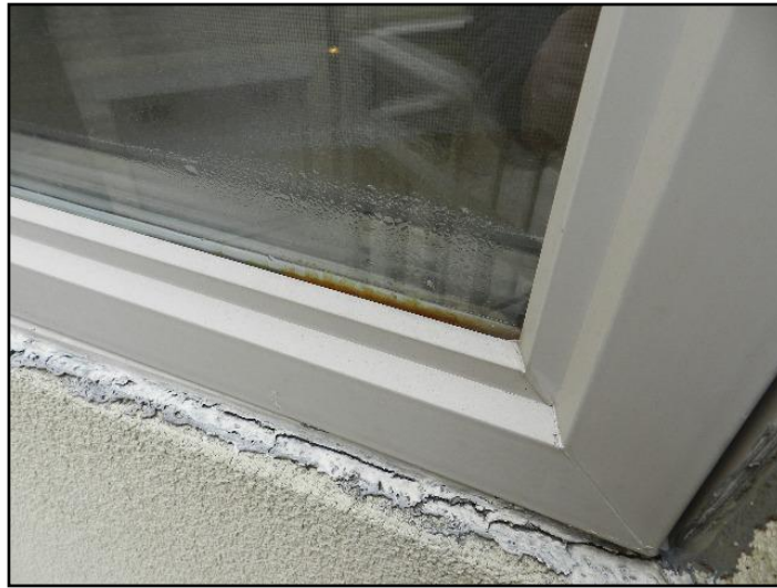
28. Excess condensation
