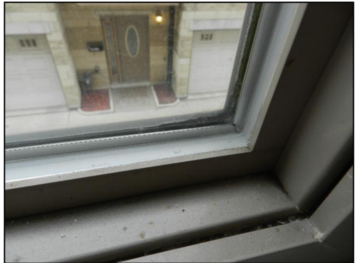
23. Lost seal on double or triple glazing
