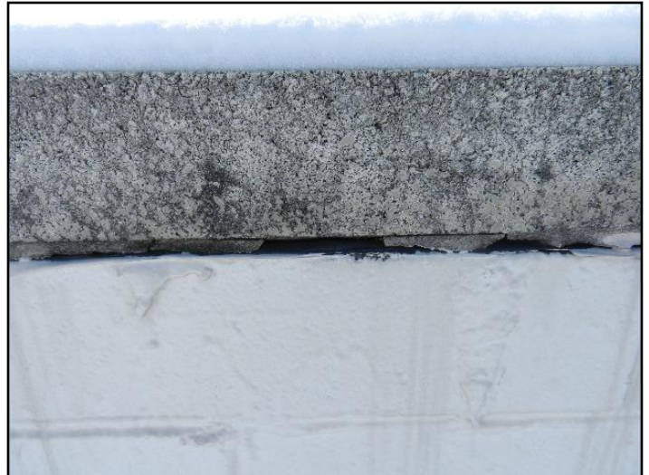
10. Inspect during annual tune-up
