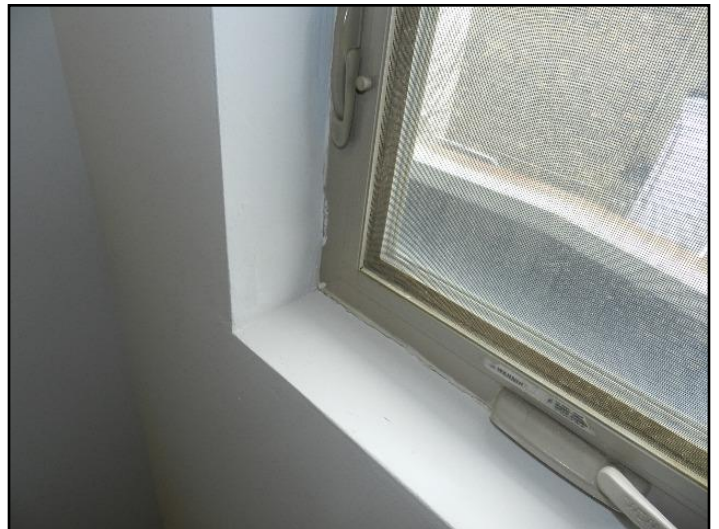
27. Lost seal on double or triple glazing
