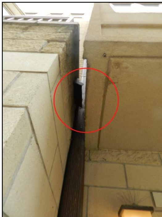
17. Discharging on a wall
