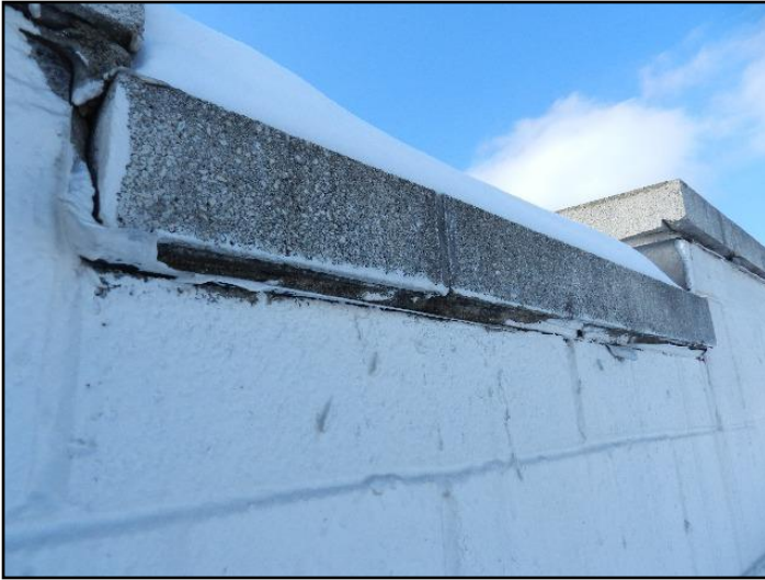
11. Inspect during annual tune-up
