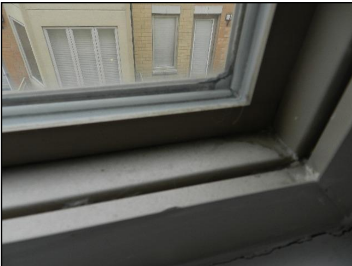
26. Lost seal on double or triple glazing
