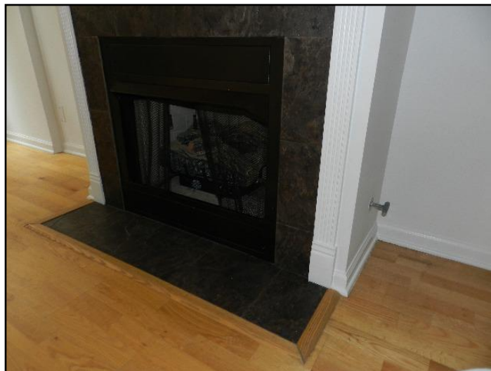
72. Unable to start the igniter
