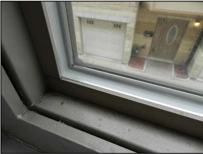
24. Lost seal on double or triple glazing
